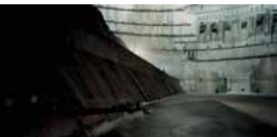
ARMIN LINKE. ReN_001318_2, Ertan Dam, Downstream Side, Panzhuhua (Sichuan), China 1998. Photographic print mounted on alu-dibond, 150 × 200 cm.
