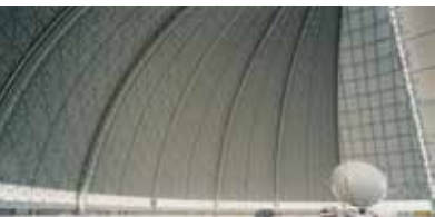
ARMIN LINKE. ReN_002986_12, Cargo Lifter for airship construction, Brandenburg (Berlin), Germany 2001. Photographic print mounted on alu-dibond, 150 × 200 cm.
